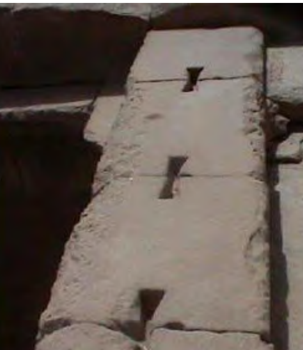
Fig. 14a. Left: Twin three-story stone pagodas, completed in 682, Unified Silla Dynasty, Gameun-sa, Gyeongju, Korea (the western pagoda in front, eastern pagoda in back). Right top: Exposed clamps on the topmost roof-stone of the eastern pagoda; Right bottom: Extracting a clamp (square-headed dumbbell type) from the western pagoda.
