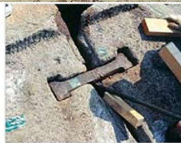
Fig. 14a. Left: Twin three-story stone pagodas, completed in 682, Unified Silla Dynasty, Gameun-sa, Gyeongju, Korea (the western pagoda in front, eastern pagoda in back). Right top: Exposed clamps on the topmost roof-stone of the eastern pagoda; Right bottom: Extracting a clamp (square-headed dumbbell type) from the western pagoda.
