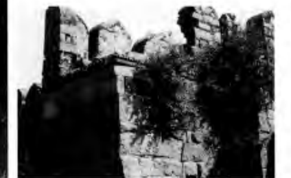
15. Muslim pointed merlons erected on the old wall/16. Square tower topped by pointed merlons.
