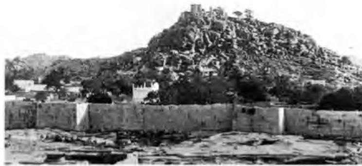
11. Raichur, curtain walls made of rectilinear segments flanked by quadrangular towers Pl. IV. Warangal (12th century) (A)
