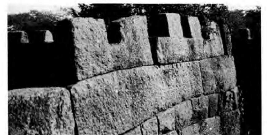
14. Parapet made of large horizontal blocks with rectangular notches.
