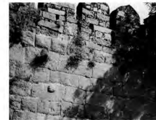
15. Muslim pointed merlons erected on the old wall/16. Square tower topped by pointed merlons.
