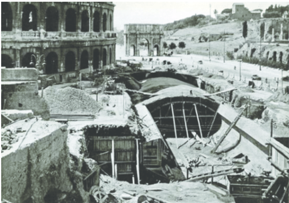
Rome-Metro-Line-B-mid-30s-Left-Excavations-right-at-the-foot-of-the-Colosseum
