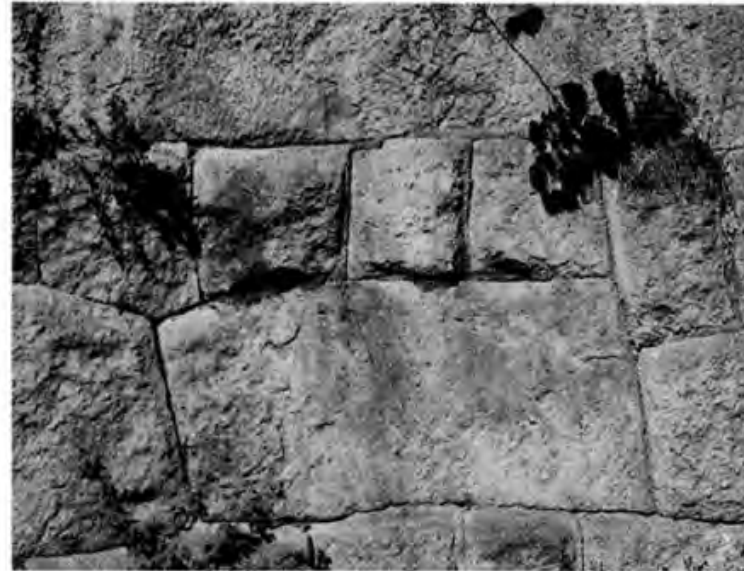
12. Granite blocks fitted closely together without mortar.
