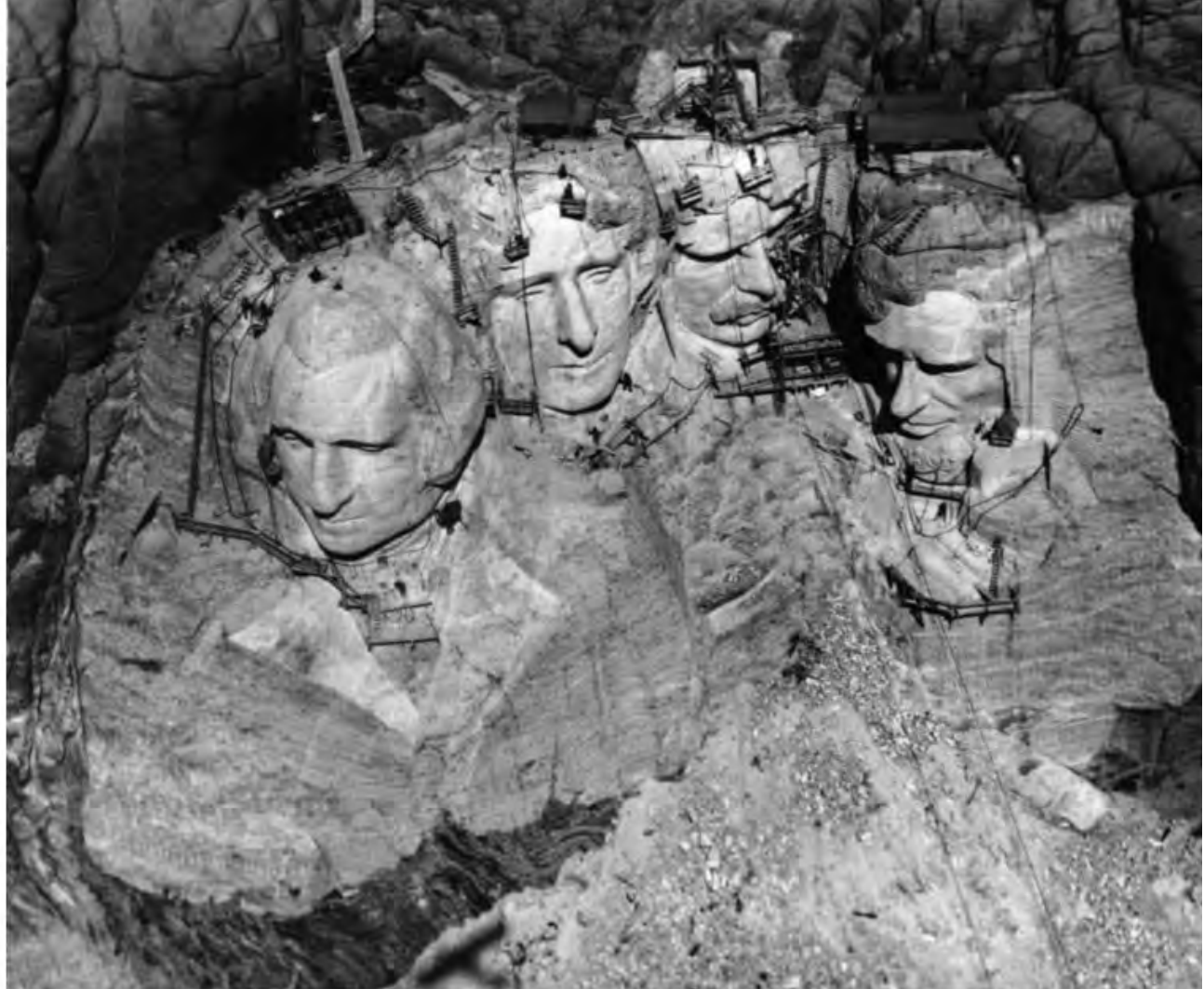
Aerial view of Mount Rushmore with many workers on the faces, scaffolding in place on top of the heads, and stairwells still in place for workers to scale the mountain | U.S. National Park Service
